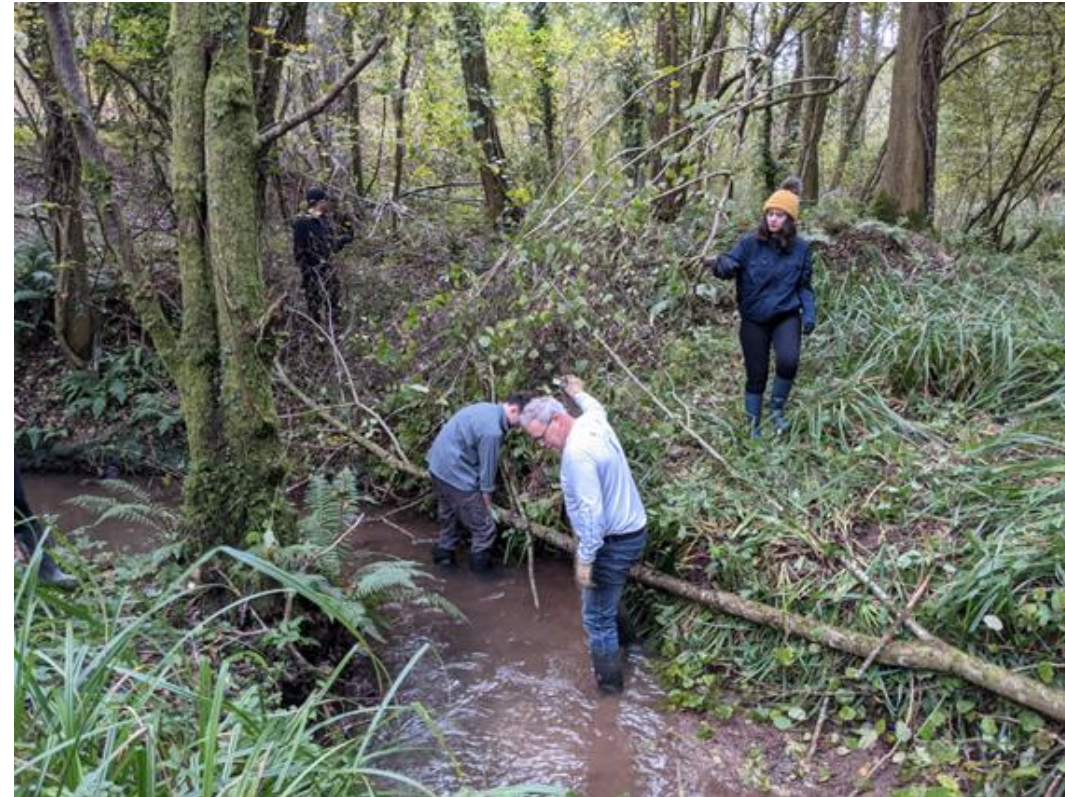
Image 19. Volunteers helped to secure the woody material in place
