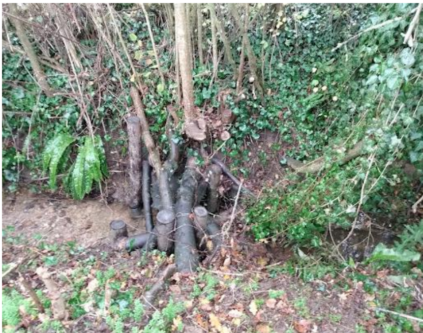
Image 11. A leaky dam was constructed along an incised tributary to slow the flow by increasing storage capacity upstream of the structure. Image credit Bristol Avon Rivers Trust
